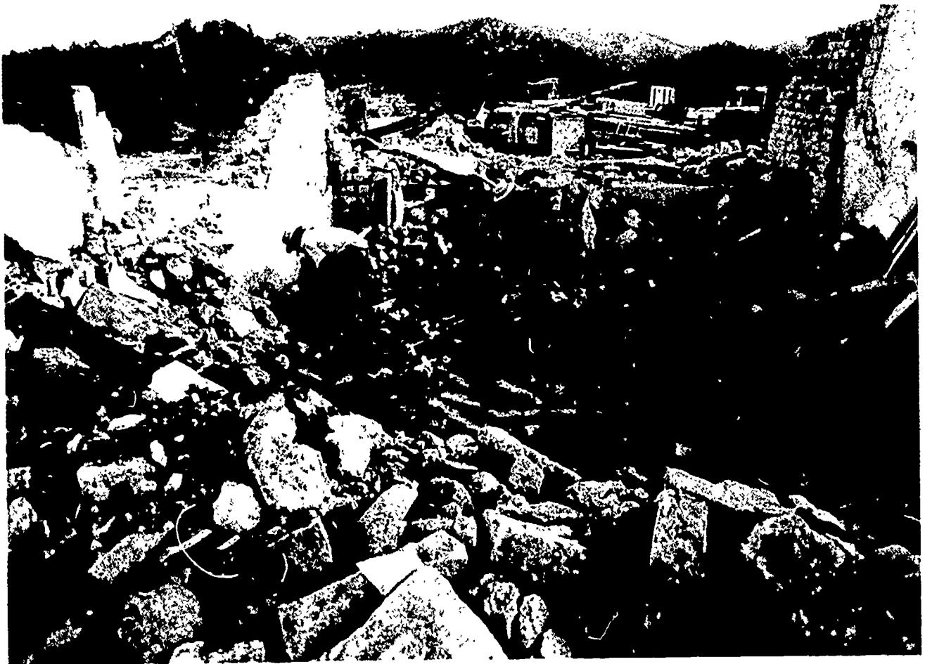
The Aftermath Of An Earthquake
